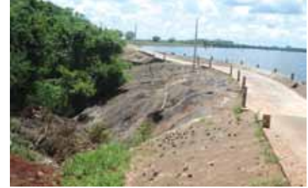
Rehabilitation Works in Progress - Kandalama Tank
