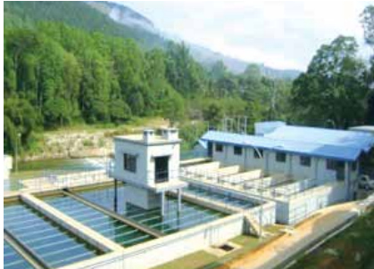
32,000m 3 /day Treatment Plant at Meewatura was constructed under the Towns South of Kandy Water Scheme.
