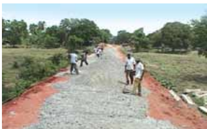
Construction of a Northern Railway Line Between Vavuniya and Omanthai
