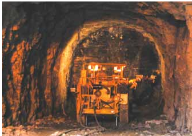
Construction of Underground Tunnel- Upper Kotmale Hydro Power Project
