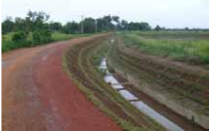
Morawewa Irrigation Scheme
