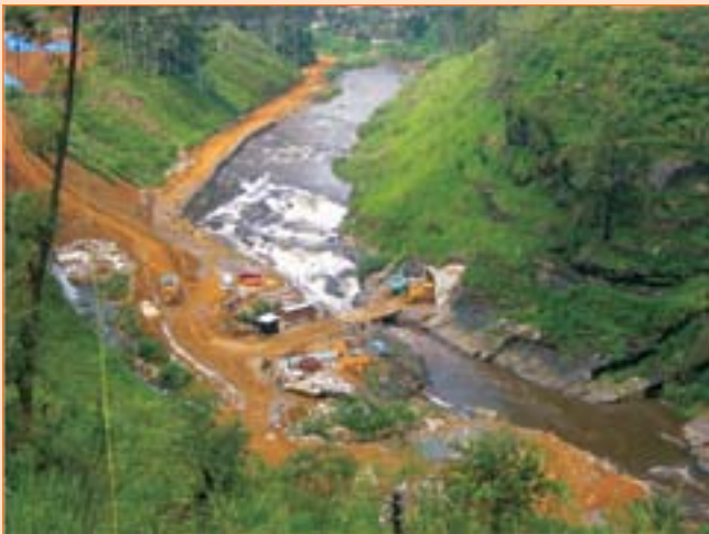
Work in Progress at Diversion Tunnel Area
