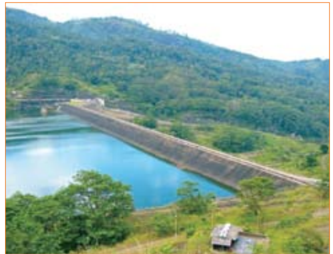
Kotmale Reservoir to be reconstructed under the Dam Safety Project.
