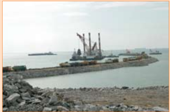
Construction of Colombo Port Breakwater
