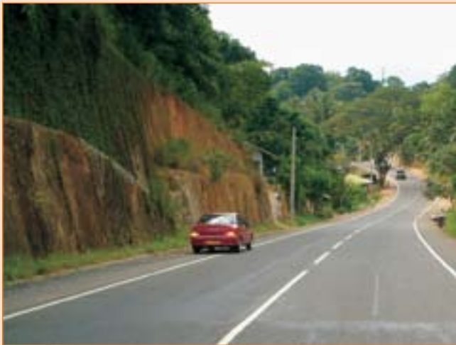
Rehabilitated Pelmadulla – Madampe Road
