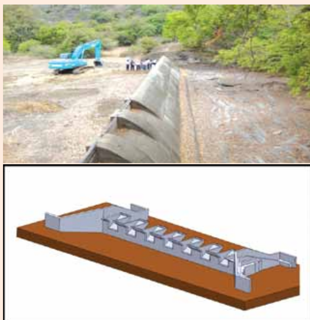
Fig 1. Giritale - Existing Spillway being replaced with a New Piano-Key Weir Type Spillway
