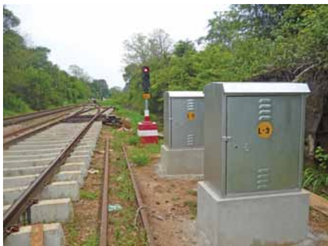
Installed Signal Boxes in Northern Railway Line
