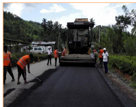
Asphalt Paving
