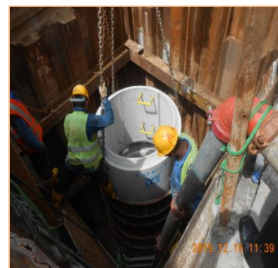
Placing a Manhole Ring of U1 sewer at Marine Drive
