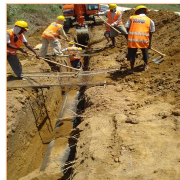
Pipe laying at Ipalogama
