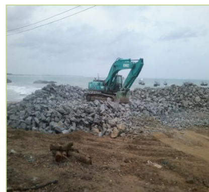
Stock piling of core material at Kalametiya Fishery Harbour
