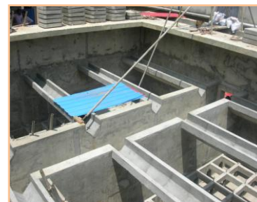
Construction of new water filter
