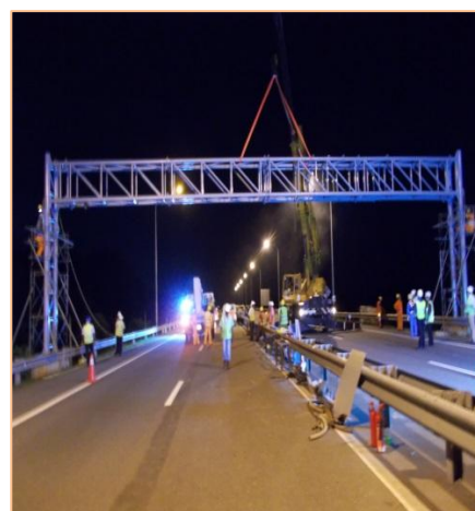
Gantry Erection
