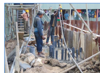
Pressure grouting to seal water seepage
