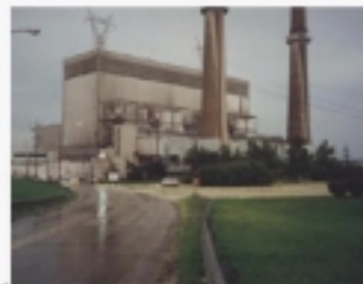
Proposed Coal Power Plant-Trincomalee
